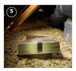
Hatch is insulated to proper R-value (the maximum R-value structurally allowable, up to the final insulation level of surrounding attic).
