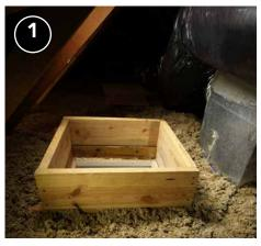
Rigid, durable damming is installed and mechanically fastened in place.
