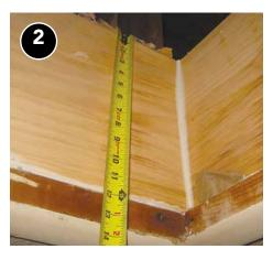
Dam is at least 2 inches taller than the final attic insulation depth.
