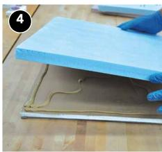
Cut and stack rigid foam insulation, gluing with appropriate adhesive, to build up R-value. Ensure the foam meets thermal or ignition barrier requirements of the authority having jurisdiction.
