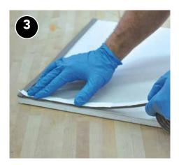
If replacement is needed, cut a gypsum or plywood board to size and use a durable weatherstrip or closed cell foam tape to create a seal.
