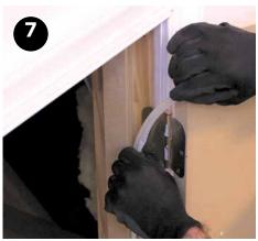
For vertical accesses, run weatherstripping or closed cell foam tape to air seal at these doorways too. Hold vertical accesses closed with latch if necessary.
