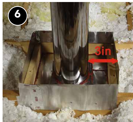
Dams are built around heat sources and air sealing is completed using approved materials (e.g., metal flashing, high-temperature rated sealants, etc.). The damming should be higher than the finished depth of any new insulation. Note that the clearance distance from damming to insulation can vary; follow guidance from the authority having jurisdiction.
