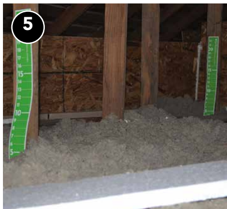
Insulation depth rulers installed, 1 per 300 square feet.
