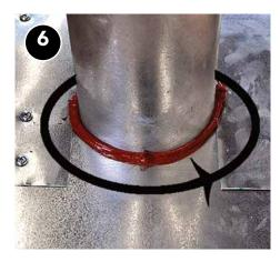
Run bead of high-temperature caulk around the chimney and seal the edge of any remaining gaps to ensure an airtight seal.
