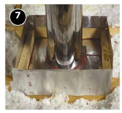
Install a durable fixed dam, at least 2 inches higher than final insulation level, keeping all combustible materials at least 3 inches away from flue or chimney.
