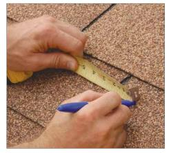
Mark out size and location of hole on roof deck, verifying size of termination collar.
