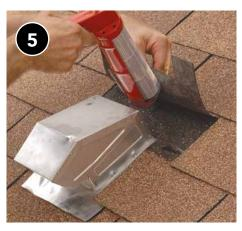
Run sealant around perimeter of vent and tuck under any surrounding uphill shingles. Seal uphill shingles over vent.
