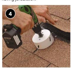
From roof side, cut hole slightly larger than termination collar. Note that when installing passive attic roof vents, a reciprocating saw is typically used.
