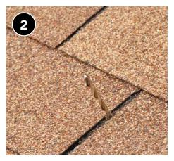
Locate the ideal location for the vent and, from the attic side of the roof, drill a small pilot hole centered between the roof rafters. Exterior exhaust terminations should be located at least 3 feet from property lines, operable openings (windows and doors) to the home, and at least 10 feet from mechanical intakes or distances specified by the authority having jurisdiction.
