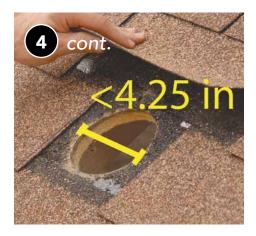
If shingle roof, cut just below one layer of shingles in order to preserve overlap.
