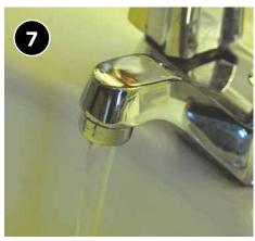
Run water through new aerator to verify it is not cross-threaded and no water is leaking around sides.
