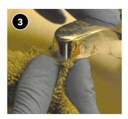
Clean threads of the faucet with a soft rag to remove any debris.
