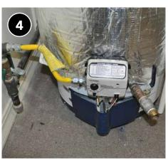
Do not obstruct burner access plate or combustion air intake.
