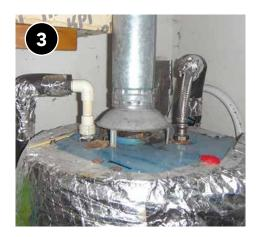
Tape insulation to the top of the water heater while maintaining a minimum clearance of 6 inches from draft diverter.
