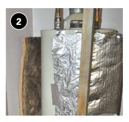
Carefully wrap the insulation around the water heater, using tape to hold the blanket together.
