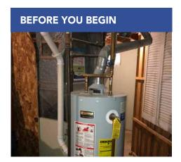
Check data plate and warning labels on water heater to find existing insulation level and confirm additional insulation is not prohibited by the manufacturer.
