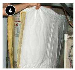
Carefully wrap the insulation around the water heater, and tape the seam and edges. Secure the insulation in place with plastic ties and avoid cinching them so tightly that the insulation is compressed.
