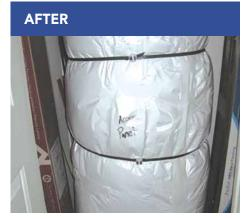
With access panel flaps cut and labeled, a properly insulated water heater reduces standby losses while allowing access to the water heater control panels.
