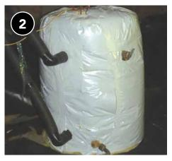
Ensure a continuous vapor barrier with no gaps and mark for cutout locations of any access panels or safety features such as the temperature and pressure relief valve.
