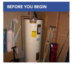
Check data plate and warning label to find existing tank insulation level and confirm additional insulation is not prohibited by the manufacturer.
