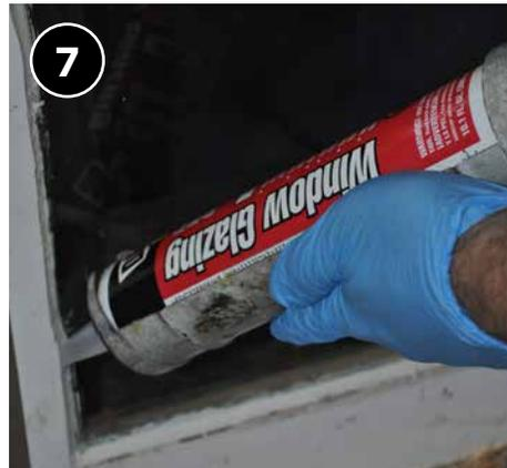
Install glazing compound or sealant at all edges of the glass.
