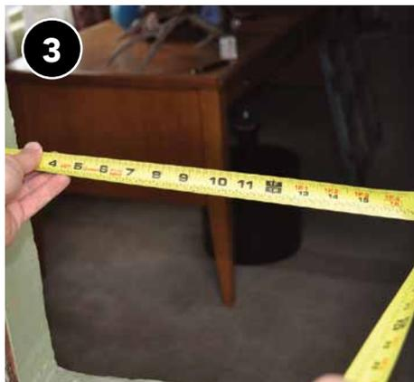
3 Measure rough opening for pane, size pane 1/8–3/16 inches smaller than the opening to ensure proper fit and minimize the potential of the glass cracking during installation.
