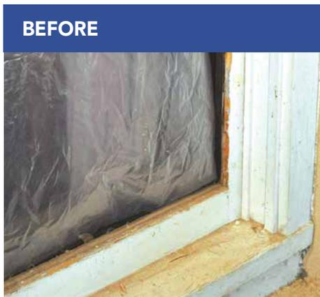
Broken, cracked, or missing glass breaks the pressure and thermal boundary.
