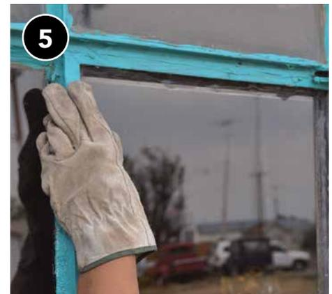
5 Install new glass, using tempered where code requires, that meets or exceeds the specifications of the previous glazing.
