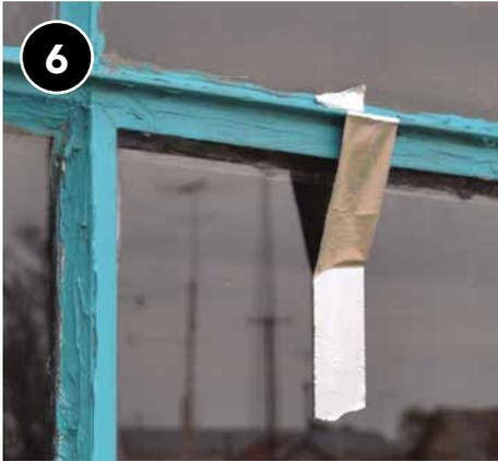
Temporarily hold new pane with tape and carefully install new push points.
