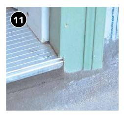
Seal along threshold, ensuring water will flow away from door.
