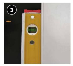
Prepare opening by ensuring that jambs are plumb and threshold is level.
