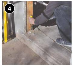
Clean, frame-in (if needed), and adjust opening as necessary to accommodate new door.
