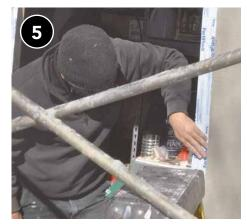
Attach flashing, if necessary, to protect any new materials from water intrusion.
