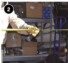
Measure opening and ensure that the door on location is the proper size.
