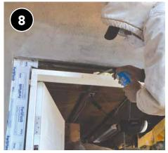
Insulate gaps between door jamb and frame.
