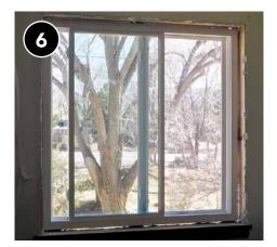
Level the window using shims
