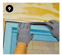
Insulate and seal rough opening with backer rod and/or low expansion spray foam.
