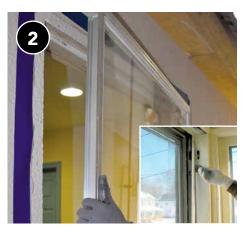
Carefully remove window trim/stops prior to removing the existing window.
