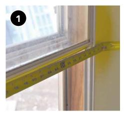
Measure window rough opening to confirm the replacement window is the correct size and will fit.
