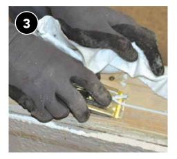
Clean up jamb and repair any damage. Insulate sash weight cavities with low expanding spray foam if present.
