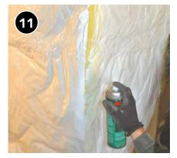
Spray adhesive along vapor retarder at seam to seal closed.
