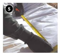
Measure insulation to take maximum advantage of large sheets of duct insulation.
