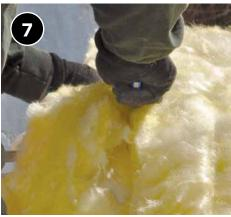
To ensure a complete vapor retarder, trim insulation from vapor barrier to create overlap flap for seams or tape seams with UL-181 tape.
