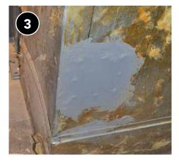
Patch holes in ducts and plenum with appropriate materials (see 19-1 Seal Ducts With Mastic).
