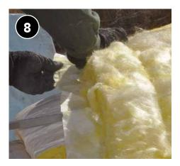
Ensure clean surface for adhesion at overlap seam.
