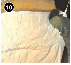
Ensure smooth and unrippled adhesion of insulation to metal of plenum.
