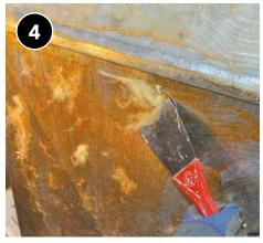
Prepare plenum by removing any residue from old insulation.
