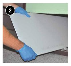
Check return cavities inside building envelope to ensure they are sealed off from unconditioned spaces.
