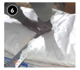
Cut to size for area to be covered. Insulate all exposed metal of the plenum.
