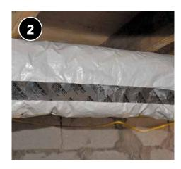
Tape joints to secure insulation in place.
