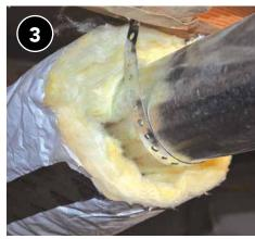
Ensure insulation is not compressed.
