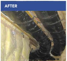
Well-supported and uniformlyinsulated ducts perform at higher efficiency.
