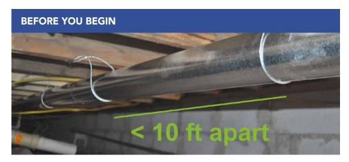
Verify ducts are properly connected, supported, and sealed.
