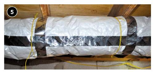
Use twine or zip ties to provide additional support, being careful to not compress the insulation.
