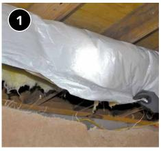
Layer insulation around duct, fitting between duct and construction members as necessary.
