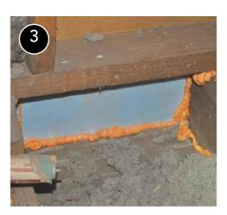
Place blocking material (sealed at edges) as needed to block open cavities and chases prior to adding insulation.
