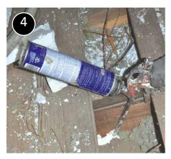
Air seal. Check for and air seal electrical, plumbing, and HVAC penetrations properly.
