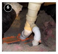
Other penetrations such as plumbing vents can be sealed using foam or caulk with backer rod as described in step 4.
