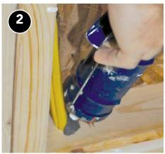
For smaller gaps, caulk is enough to seal the hole.
