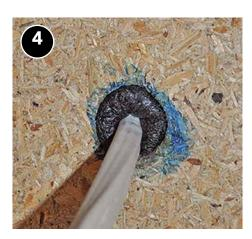
Inserting backer rod provides infill to support the sealant.
