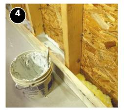
Securely fasten rigid material capable of withstanding air pressure if the wall cavities will be dense-packed.
