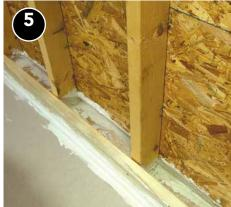
Seal any remaining gaps with caulk, one-part foam, or mastic. Extend the sealant to adjacent materials.
