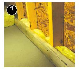
Block the opening of balloon framed sidewalls in alignment with the pressure boundary.
