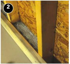
Blocking material options include lumber, gypsum board, XPS [extruded polystyrene], or bagged fiberglass batts.
