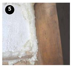
Extend sealing to adjacent materials to ensure a complete air seal.
