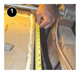
Measure the opening of the chase in a location that will maintain the pressure plane.
