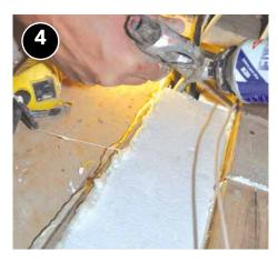
Seal all edges with caulk, spray foam, or mastic.
