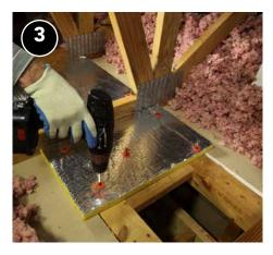
Apply sealant along top plates, bracing, and framing members prior to attaching rigid material and secure in place with mechanical fasteners.
