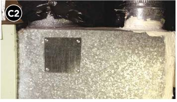
Cut patch that will extend over entire gap or hole and affix with mechanical fasteners.
