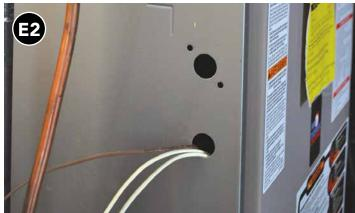
Seal unnecessary holes in air handler cabinet with UL-listed butyl tape.
