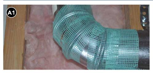
Apply fiberglass mesh tape over all gaps, seams, joints, etc.
