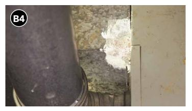
Push fiberglass mesh into the mastic.
