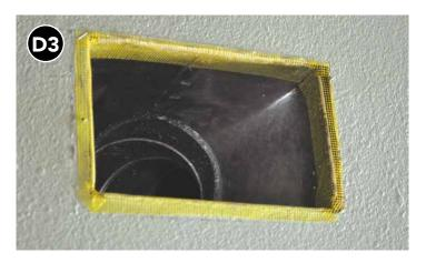
Apply fiberglass mesh tape bridging from duct boot interior to surface, taking care not to extend past what will be covered by register.
