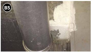
Apply additional mastic over mesh and tape, extending at least 1 inch past edges of tape in all directions.
