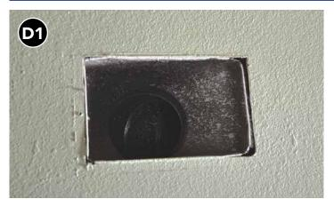
Often, holes for duct boots are cut too large and leave gaps around the boot that permit air leakage.
