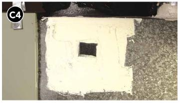
Apply additional mastic over mesh, extending at least 1 inch past tape and seam in all directions.
