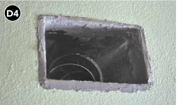
Apply mastic over mesh tape and allow to dry completely before reinstalling register.
