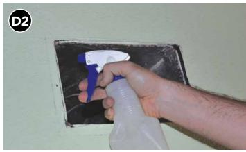
Clean the area around the duct boot to allow for better adhesion of fiberglass mesh tape.
