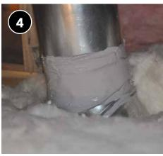
Cover mesh with a layer of mastic to seal all joints. Alternatively, the seams can be sealed with UL-listed foil tape.
