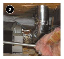
Keep duct run as short as possible with few turns, and run to exterior, either via roof or sidewall.
