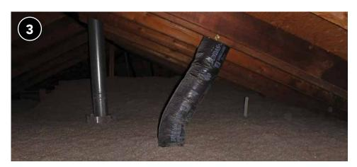
Create the shortest run possible to an exterior termination and provide adequate support as needed without compressing the duct. Ducting that runs through unconditioned spaces must be insulated.
