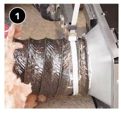
Ensure proper connection of duct to bath fan. The size of the ducting should be equal to or larger than the outlet (no downsizing or reducers).
