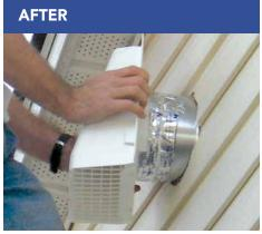
Bath fans must exhaust to the exterior of the home. Follow the manufacturer's installation instructions when installing the vent hood to ensure a water tight land durable install.
