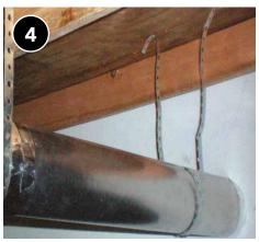
Duct terminates to outside, at a downward slope when possible.
