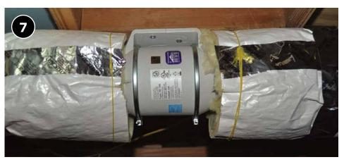
If duct run must exceed 35 feet, install booster fan.
