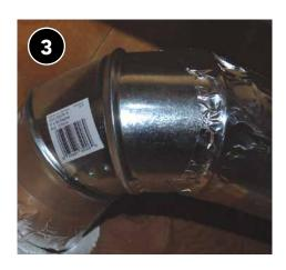
Use correct fasteners (no screws penetrating into duct).
