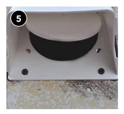
Termination has backdraft damper and no cage.
