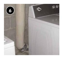
Duct in unconditioned space is insulated.
