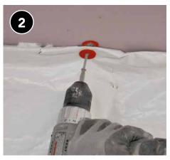
Mechanically fasten belly repair material. Seal all seams and edges.
