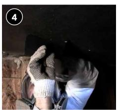
Cut access holes to ensure entire cavity will receive continuous and consistent insulation.
