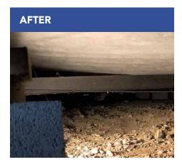
Manufactured home bellies that are insulated with complete coverage with durable repairs improve the overall efficiency of the floor assembly.
