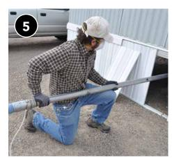
Fill entire belly cavity to prescribed R-value while ensuring plumbing has sufficient insulation value to prevent condensation or freezing.
