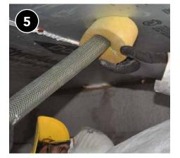
Use appropriate fill tube to insulate each cavity and ensure complete coverage.
