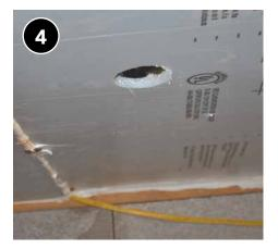
Cut an access hole into each cavity of the floor, large enough for fill tube.
