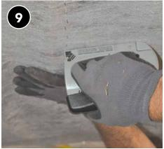
For work orders that require netting, secure a smooth layer of netting across the bottom of floor joists.
