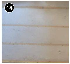
Insulation with complete coverage that does not settle will improve the thermal performance of the floor assembly.
