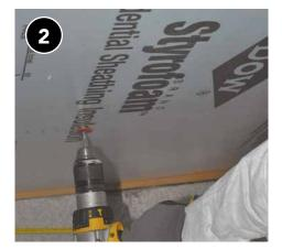
Attach rigid barrier to cover all floor cavities.
