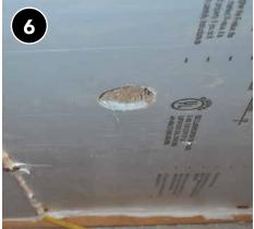
Fill cavity completely to density required by work order.
