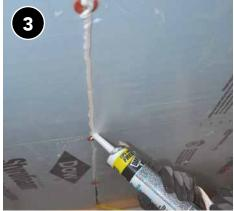
Seal seams between sheets of rigid material to prevent air movement and insulation leakage.
