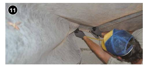
Cover the entire cavity to ensure continuous insulation coverage and prevent insulation from blowing out the ends.
