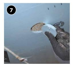
Plug access hole either with original material cut out or appropriate replacement.
