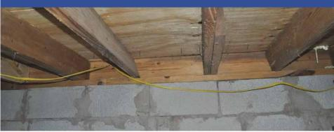
Uninsulated floor cavities present opportunities to increase the thermal performance of floors above unconditioned spaces. Insulation can be blown if a rigid barrier or netting is attached to the bottom of the floor joists.
