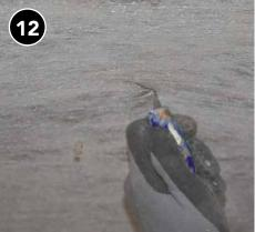
Cut access hole for fill tube.
