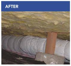
Insulation with complete coverage in contact with the subfloor will improve the thermal performance of the floor assembly.
