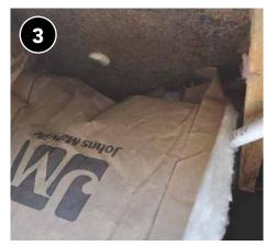
Install batts with vapor retarders so that the vapor retarder faces the conditioned space.
