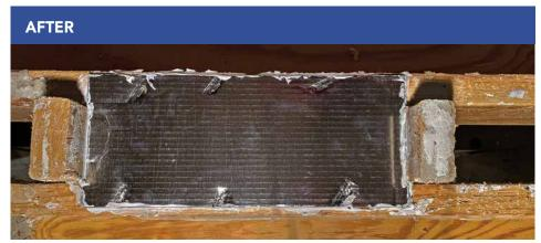
Securely sealing off these cavities prevents air movement, as well as providing a barrier to hold in insulation and providing fire blocking.
