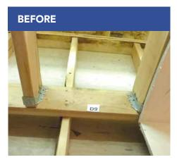
Balloon-framed walls have an open cavity that runs from the basement to the attic, allowing for large amounts of air flow via the stack effect.
