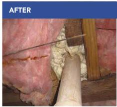
Depending on the size of the gap, one-part spray foam or a combination of infill material and foam or caulk can be used.
