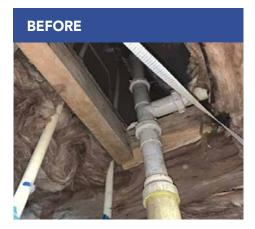
Larger penetrations in the subfloor, especially plumbing chases, need to be air sealed when they define the pressure boundary.
