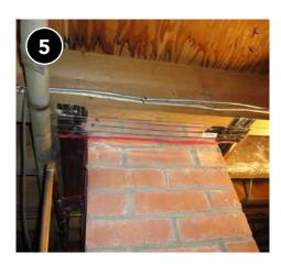
Use appropriate materials for high-temperature locations, such as around flues and chimneys.
