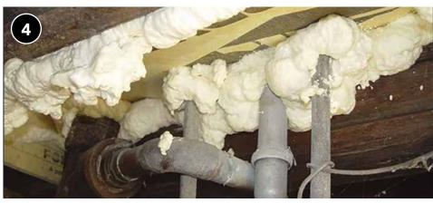
Secure rigid infill in place and seal smaller gaps around infill with appropriate materials.
