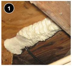
Spray foam expands to fill large holes, but may need fire protection (e.g., thermal/ignition barrier).
