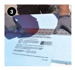
Cut rigid infill with attention to locations of pipes and electrical.
