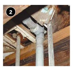
For larger holes, rigid infill material is needed.
