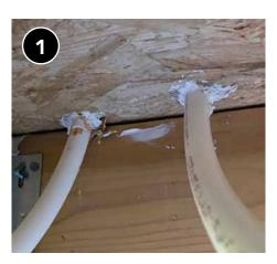
For small penetrations, caulk or sealant is often enough to seal the gap.
