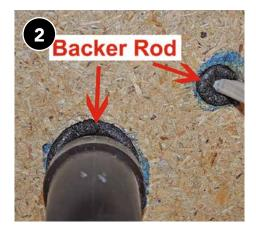
Use a backer rod or other infill material when sealing a gap larger than 1/4 inch with caulk.
