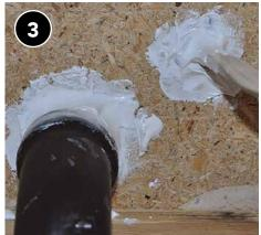
Seal over the backer rod to establish the air seal.
