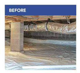
Unvented crawl spaces are sometimes considered to be part of the conditioned space, so the walls need insulation.
