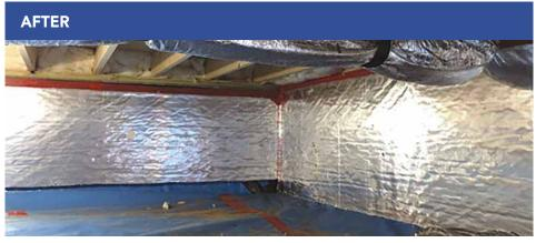
Insulation is or has class II vapor retarder facing conditioned space. Insulation laps underneath ground vapor retarder at foundation wall.
