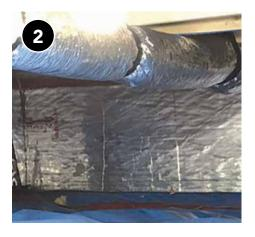
Attach insulation in a durable manner and seal seams and edges with compatible materials.
