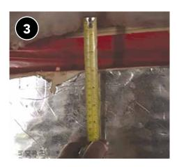
Leave a 3-inch termite inspection gap between the bottom of the sill plate at the top of the insulation, if required.
