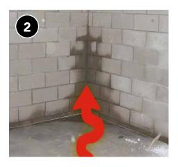
Check wall for water intrusion that needs to be mitigated first. All bulk sources of moisture should be directed away from the foundation walls.
