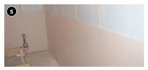
Install a sealed air barrier on the conditioned side of the insulation. When using foam, gypsum board must be at least 1/2 inch to meet building code requirements as a thermal barrier.
