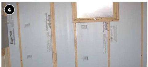
Install insulation using mechanical fasteners to prescribed R-value in full contact with the entire perimeter of the foundation wall from ceiling to floor.
