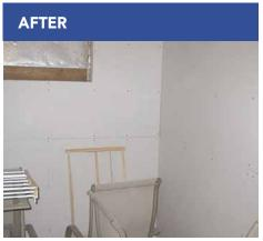
A sealed continuous air barrier finishes off an insulated basement wall, providing air sealing benefits and improved thermal comfort while reducing heat transfer of the wall assembly.
