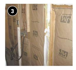
If insulation has vapor retarder on only one side, install the facing towards the conditioned space.
