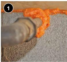
Check the foundation wall for penetrations and air seal as needed prior to installing insulation.
