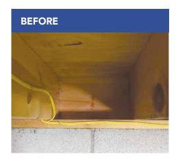
Basement and crawl space rim joists should be insulated when they define the thermal boundary.
