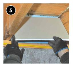
If foam insulation is more than 3.25 inches thick or space is permanently habitable, insulation needs to be covered by a thermal barrier, such as gypsum board. If requirements vary from this practice in your area, consult local code officials for clarification.
