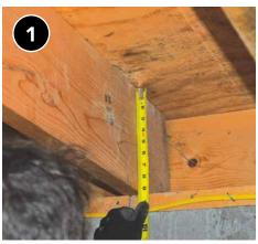
Measure each individual cavity to be insulated and take note of obstacles where insulation needs to be trimmed for a proper fit.
