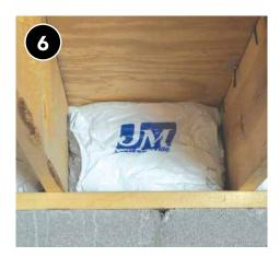
When using wrapped or faced batts, ensure facing is to the conditioned side and ensure the cavity is air sealed before installing the insulation.
