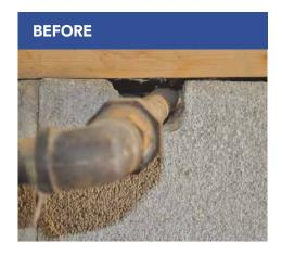
Air movement around sill plates and near rim joists needs to be addressed before insulating.
