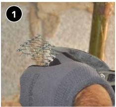
For exterior holes larger than 1/4 inch, use steel wool or other pest blocking material before sealing.
