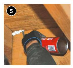
Push sealant into seams where framing members meet while installing a continuous bead around all four sides of the pocket including any gaps in the sill plate.
