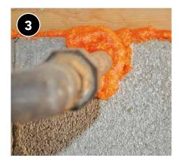
Install sealant to hold backing material in place and air seal.
