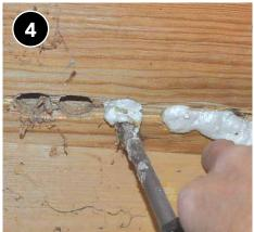
Seal penetrations (electrical, plumbing, empty holes, etc.) at the subfloor that are located within the rim joist pocket.
