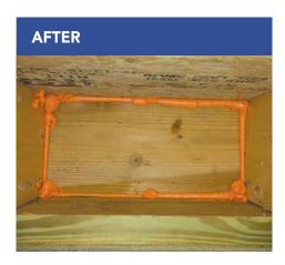
A continuous seal is achieved and the pocket is ready for insulation. Note: if using two-part foam to air seal and insulate, step 5 can be accomplished by spraying the outer edges of the pocket using a picture frame technique, then working towards the inside of the cavity to insulate.
