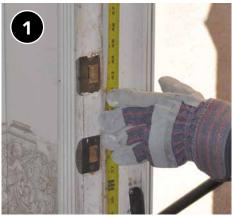
Measure each side of the doorway to determine the size of the weatherstripping.
