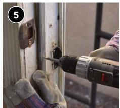
Fasten weatherstripping securely using short screws provided by the manufacturer. Check the door for smooth operation and make any necessary adjustments.
