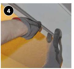
Fit weatherstripping snuggly into place after applying a thin bead of caulk that aligns with the screw holes on the backside of the weatherstripping.
