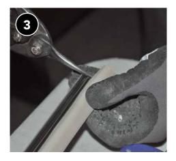
Notch the ends of each side piece of weatherstripping to allow for a tight fit with the top piece if a notch is not provided from the manufacturer.
