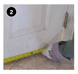
Measure door top or bottom as well for weatherstripping and potential door bottom or sweep.
