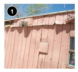
Ensure the integrity of the wall to be insulated, both from exterior and interior. Note: This home is not suitable for wall insulation as the exterior does not keep water out and the cladding is damaged beyond basic repair.
