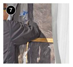
Gently tug batt into place, tuck remaining batt under lower belt rail, and fit down to bottom of cavity with minimal compression.
