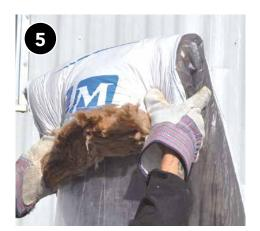
Fold the batt over the insulation stuffing tool.
