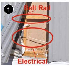
Remove siding as needed, starting from the bottom and taking note of any obstacles that may compress insulation.
