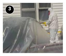
Close all doors and windows within 20 feet of the work area. Note that doors used as entrances to the work area should be covered with plastic sheeting that allows workers to pass through while containing the spread of dust.
