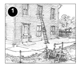
Create containment area with plastic sheeting 10 feet in any direction from work area and use barrier tape to define a perimeter 20 feet from work area to prevent unauthorized personnel from entering.
