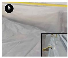
Tape plastic up onto work surface and utilize systems to catch debris while limiting damage to exterior plantings.
