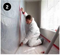
Use disposable physical barriers to mark out and contain work area dust and debris. Cover access doorways within the work area using two pieces of plastic sheeting.
