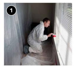
Move all objects out of work area or cover with plastic sheeting. Seal all edges and seams.
