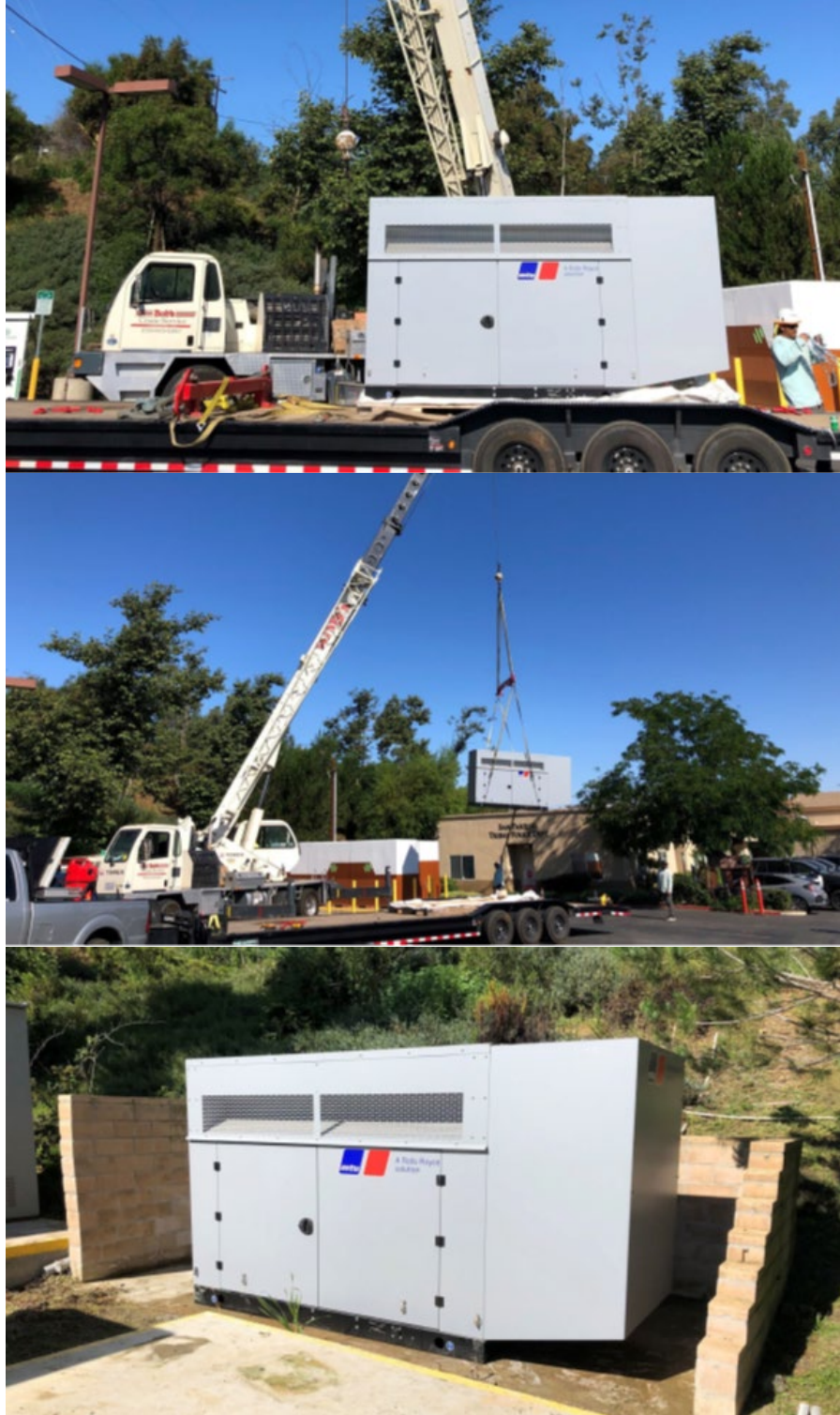
Image 4: From top to bottom: liquid propane genset delivery; lifting the genset in place; genset installed.
