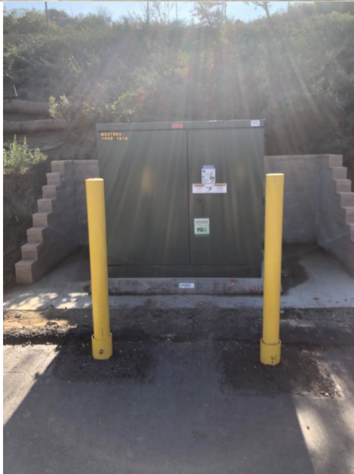
Image 3: Pad ready for transformer (top), and installed transformer (bottom).
