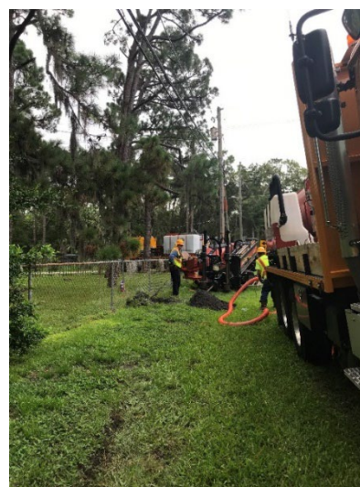
Figure 1. Left: A utility pole was downed in Florida as Hurricane Irma passed through Duke Energy Florida's service area. Right: Duke Energy Florida contractors working to strengthen the grid by installing underground lines.
