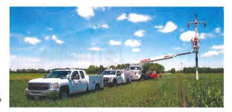
A boom truck lifts a Minnkota lineworker up to install blink outage mitigation equipment on a 69-kV transmission structure near Larimore, N.D. This program has helped significantly reduce momentary outages across the system.
