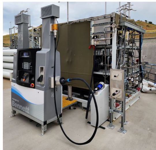
Heavy-Duty Dispenser Systems Installed at NREL's HD R&D Station (2023)
