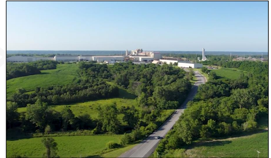
SSAB mill, located in Montpelier, IA
