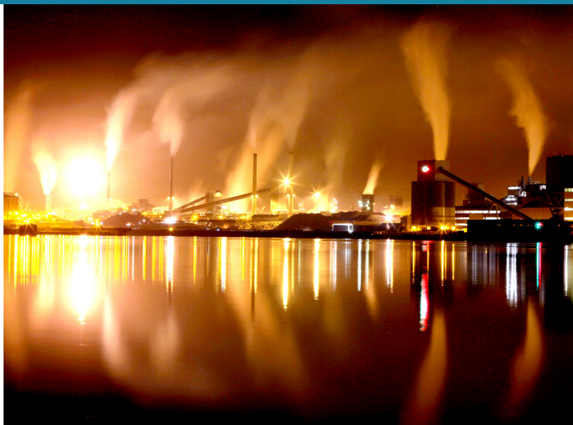
Tata Steel IJmuiden, the Netherlands. Image Credit: Joost J. Bakker, CC BY 2.0.
