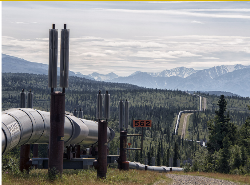
Alaskan oil pipeline, image by Gillfoto, CC-BY-SA-4.0.
