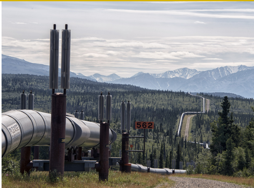
Alaskan oil pipeline, image by Gillfoto, CC-BY-SA-4.0.
