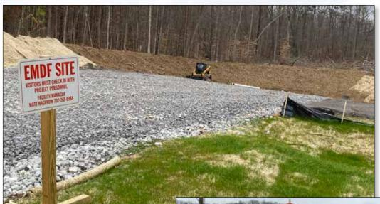
Left: Early site preparation for EMDF is expected to be complete this spring. The second construction phase will include a groundwater field demonstration study located on a portion of the final footprint of the site. Oak Ridge will gather data for two wet seasons to inform final design choices for the facility.
