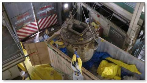
Workers in the Oak Ridge Research Reactor facility remove the top portion of the reactor vessel for disposal. They will remove the next portion of the reactor vessel this year.
