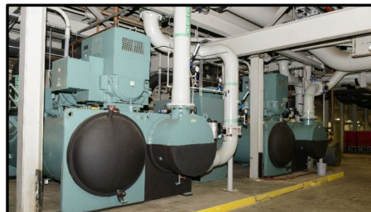
New Trane Chiller not needing R-123 Image Credit: Y-12
