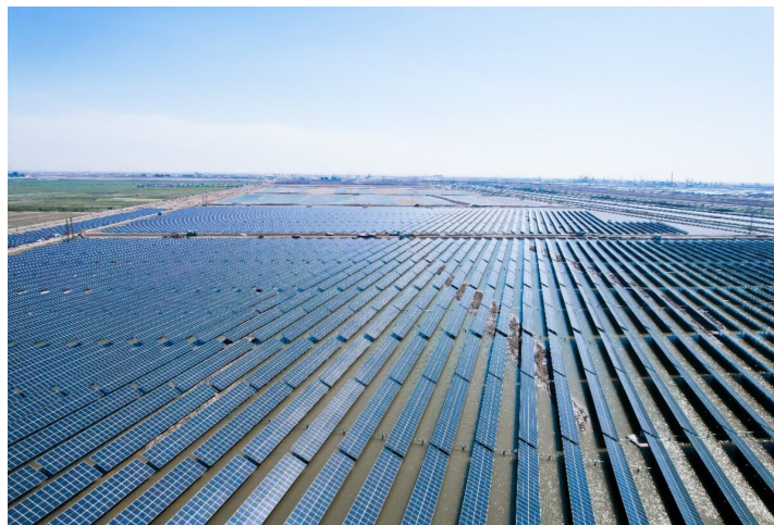
Trina Solar's modules in a 70 MW fishery PV project
