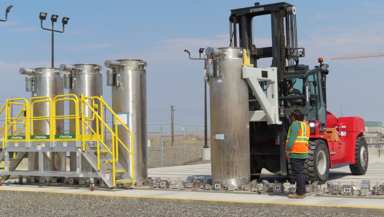
Workers move ion exchange columns filled with radioactive cesium and solids from the TSCR System on a storage pad.
