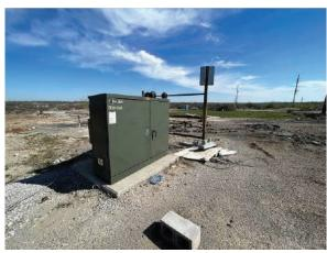
Photo #31 Pad mounted electrical transformer for former IDecker plant
