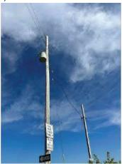
Photo #28 Facing E: Pole mounted electrical transformer, E end of former IDecker plant
