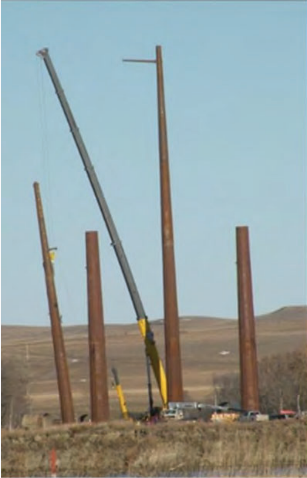
Figure B-6. Example tangent structure under construction, similar to the proposed structure at the river crossing.
