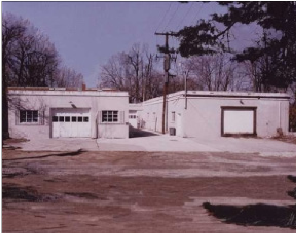
Figure 25-2. The Alba Craft Laboratory Building Before Remediation (DOE Digital Archive)
