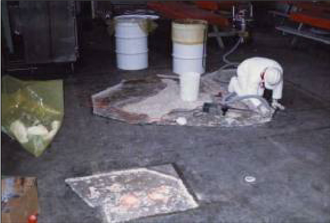
Figure 11-3. Scabbling Concrete at the Chicago North Site (DOE Digital Archive)
