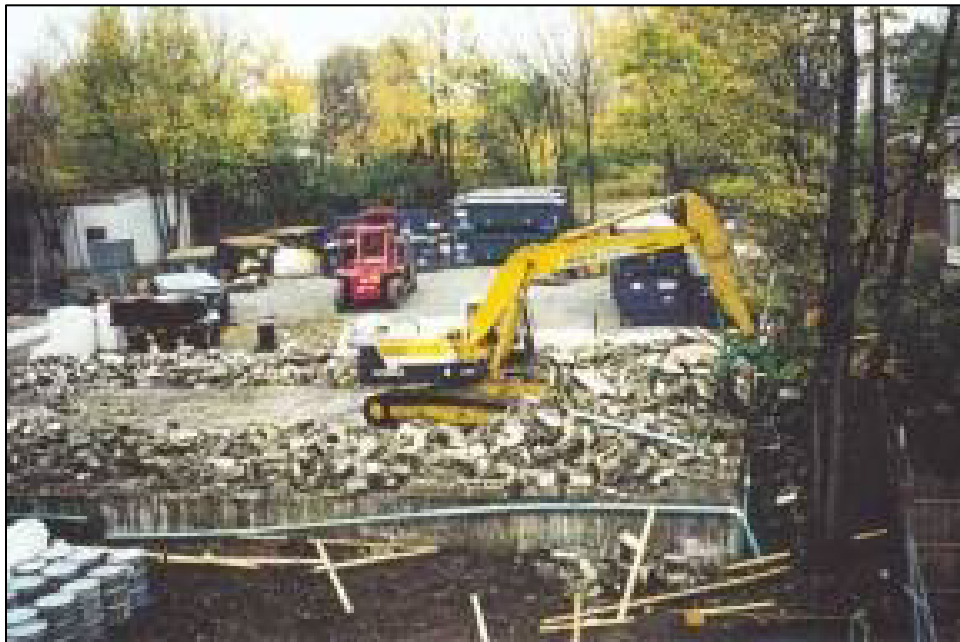
Figure 25-3. Demolition of the Alba Craft Laboratory Building, October 1994 (DOE Digital Archive)
