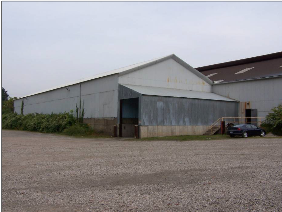
Figure 5-2. Front of Remediated Building Where AEC Work Occurred, Aliquippa, Pennsylvania, Site, September 2005
