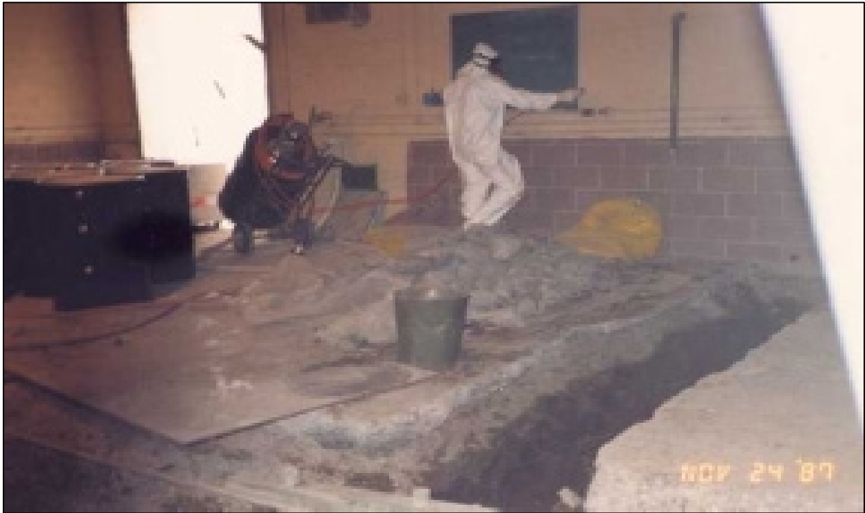
Figure 4-2. Scrubbing and Sanding at Building 31, Albany, Oregon, Site (DOE Digital Archive)
