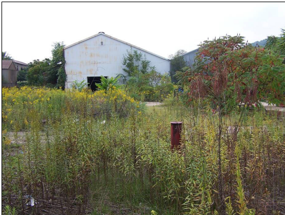
Figure 5-3. Rear of Remediated Building, Aliquippa, Pennsylvania, Site, September 2005
