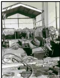
The vessel and concrete are removed.
