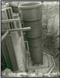
The containment vessel is put in place.
